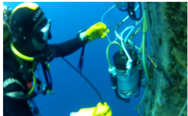
A diver working to install the pCO2 sensor along the buoy's hull.
